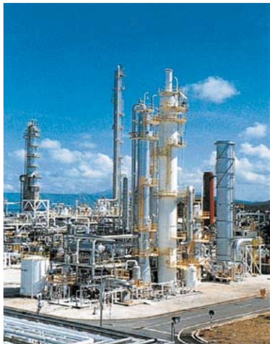
Figure 3.5 \text{CO}_2 capture plant in Malaysia using a 200 \text{ tonne d}^{-1} KEPSCO/MHI chemical solvent process (Courtesy of Mitsubishi).
